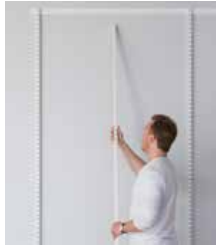
Screw the Top track into the wall.
