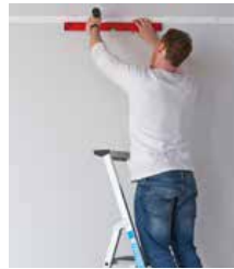
Hang the hang standards on the Top track.
